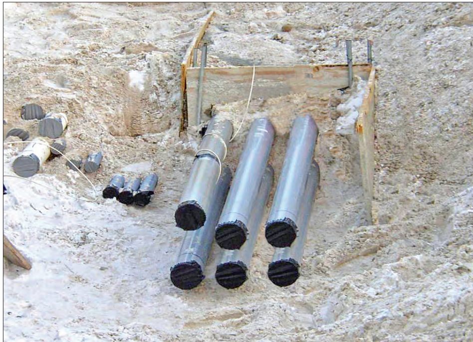
Duct work for equivalent 1000' of 1000 KCM copper conductor (1 circuit) underground with neutral - $105,000 (no duct work cost included)
