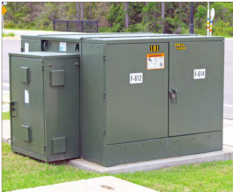
Equivalent underground three-phase switch - $80,400 (no base)
