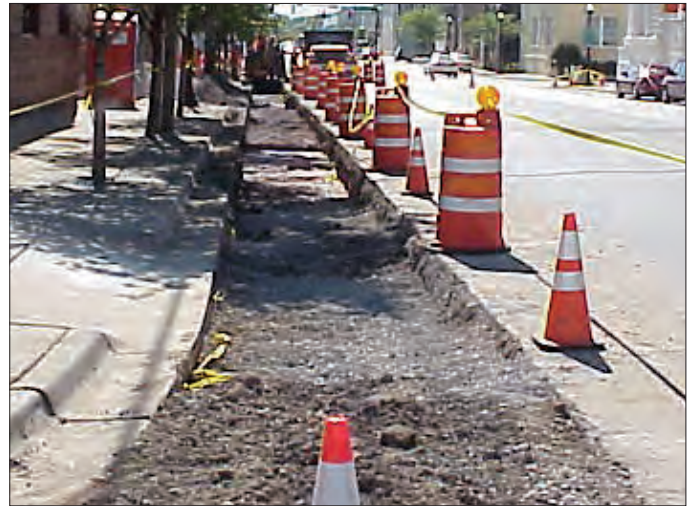
The utility easement for Pensacola's Main Street conversion is along the curb in the parking lane.
