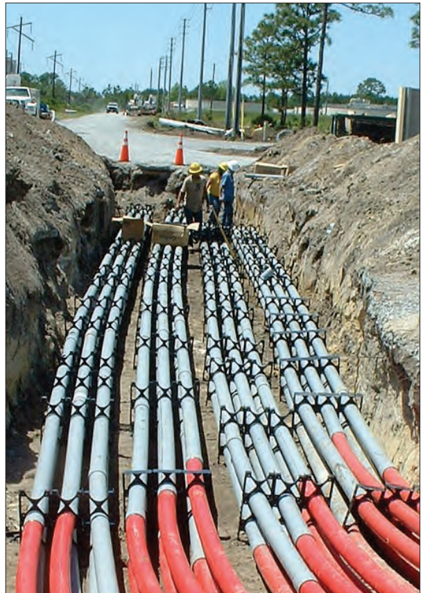
Four feeders near a substation require a large construction footprint
