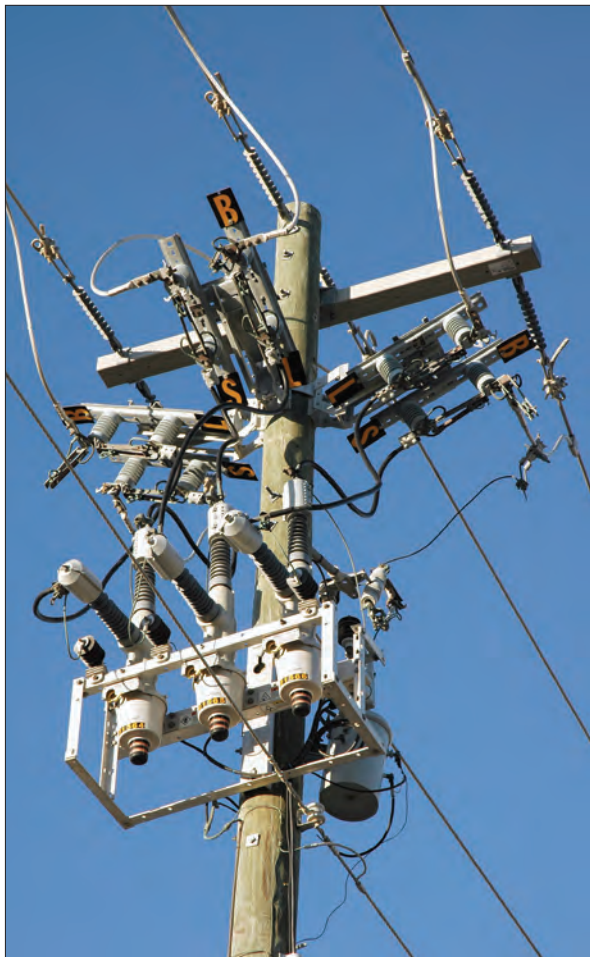
Overhead three-phase recloser - $24,400 (no pole)
