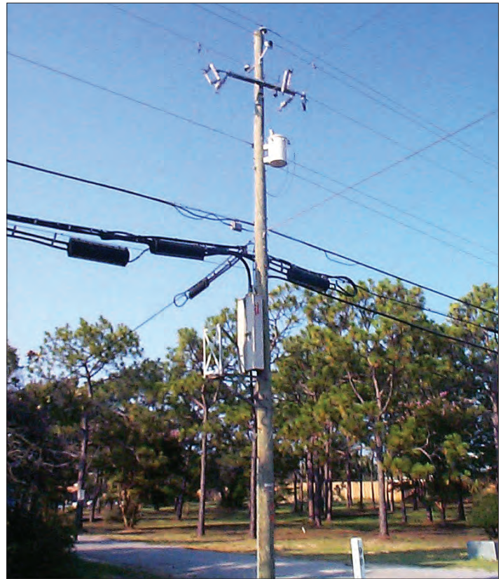
This wooden pole carries electric, cable television and telephone lines as well as an electric transformer and telephone junction box and platform.
