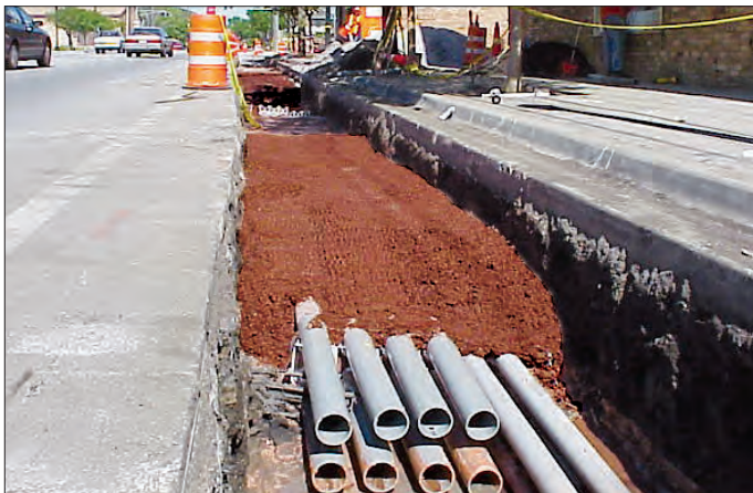
Pensacola Main Street during construction. Optional red tinted concrete marks the location of underground utilities.
