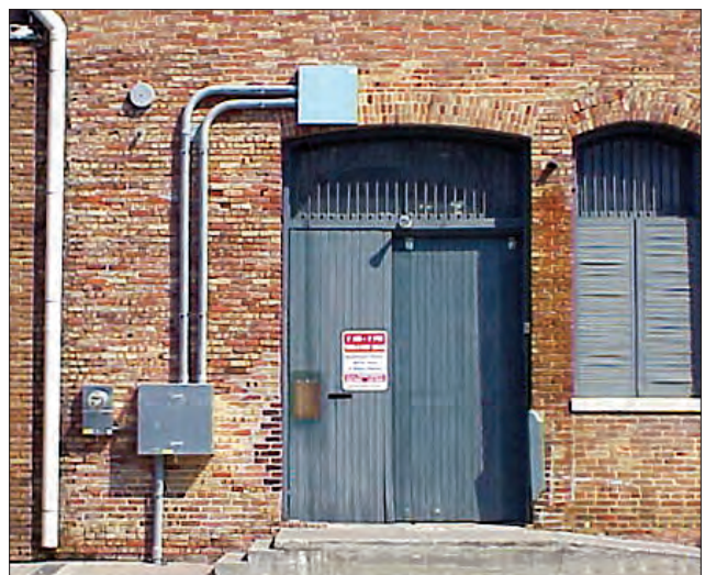
Underground service entrance upon completion of the Main Street project.
