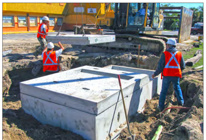
A concrete vault for switch gear requires larger easements.
