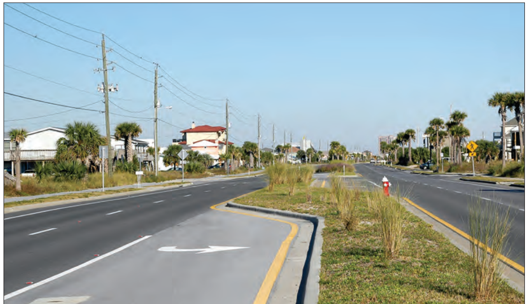
Mainline feeder system with no overhead crossovers on Pensacola Beach.
