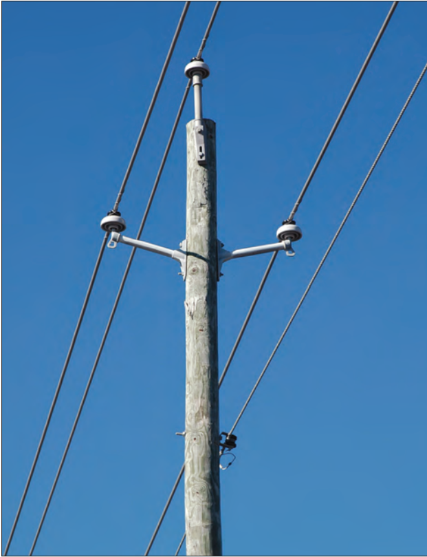
Overhead three-phase 795 AAC construction. 1000 feet of 795 AAC overhead conductor with neutral - $4,500 (no poles or hardware)
