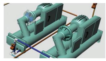
It's important to select a chiller (and its associated efficiency) carefully. Choosing a chiller that's most efficient at full or part load, according to standard ratings, might be counterproductive because the ratings don't measure the efficiency of the overall cooling system. An analysis of the entire chiller plant, preferably using simulations, will tell whether a more efficient chiller is a better option than upgrading the auxiliary equipment or improving operating strategies.
